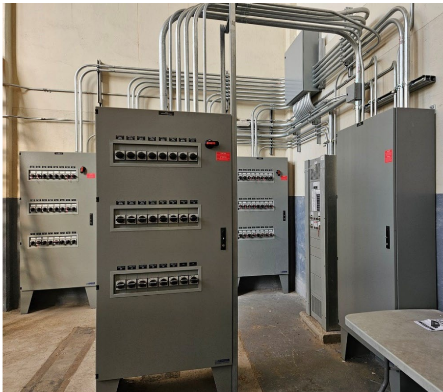
PLC panels for Bin Automation System
